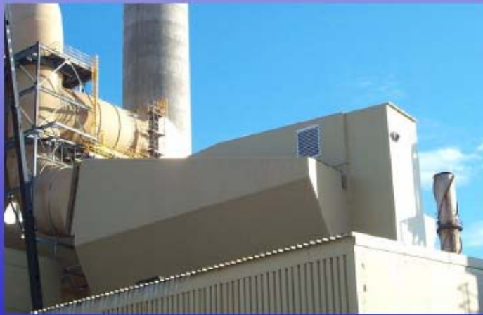
Wet Electrostatic Precipitators
