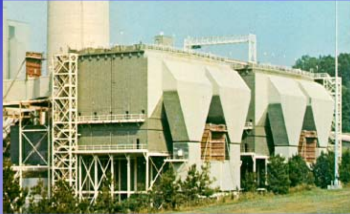
Wet Electrostatic Precipitators
